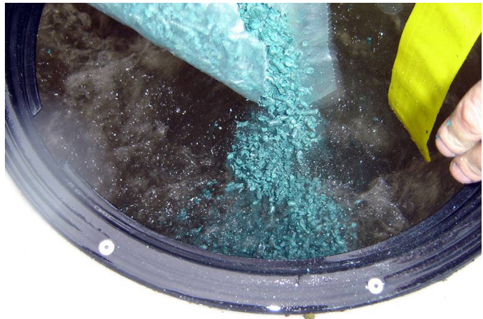
Mixing components for hydroseeding
