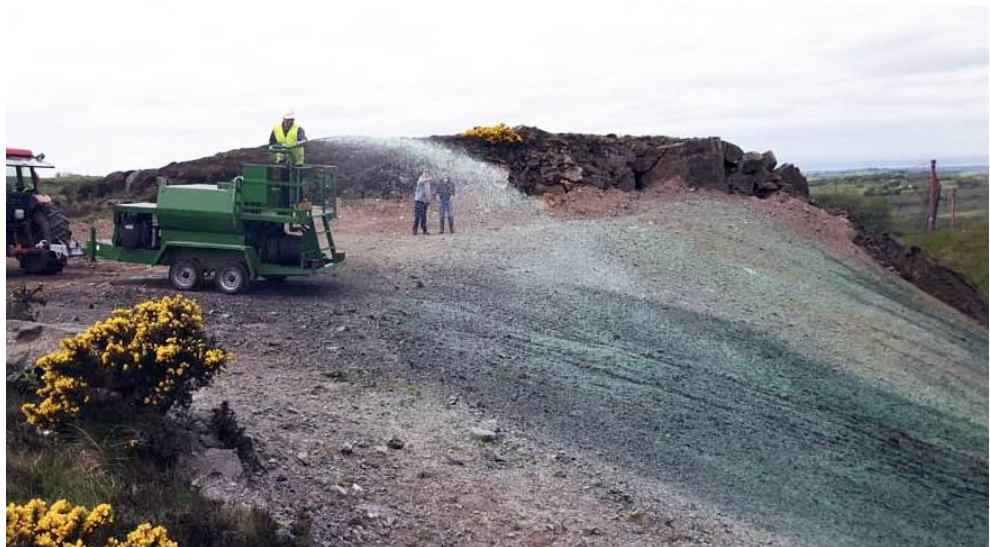
2,500 litre hydroseeder sowing steep sloping area
