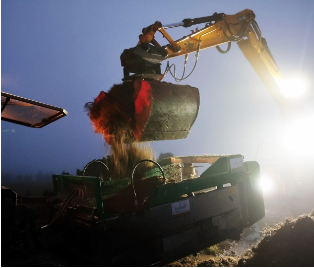
Transferring brush to spreader, Murley Mountain Wind Farm, Tyrone
